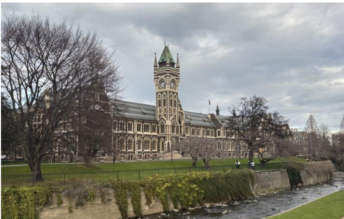
Univ. of Otago Registry Building, Dunedin, New Zealand
